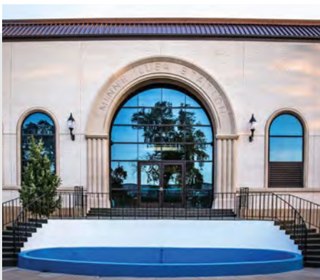
Florence Water Treatment Plant
