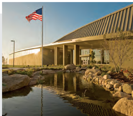
Platte West Water Treatment Plant
